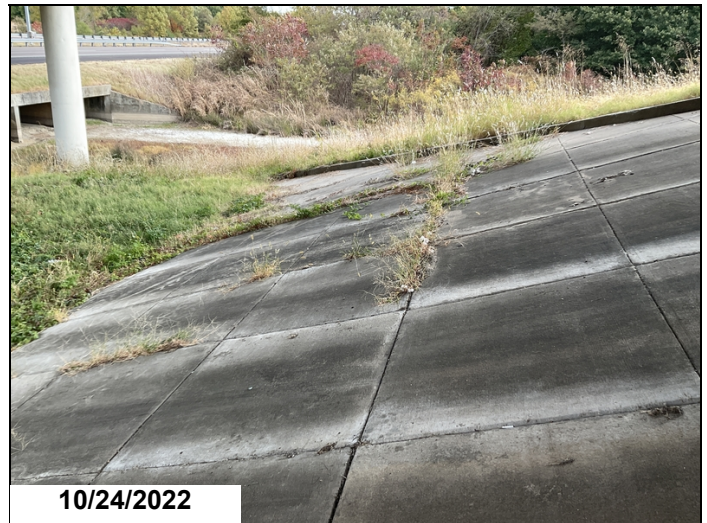
Vegetation growing in slope pavement joints abutment #1
