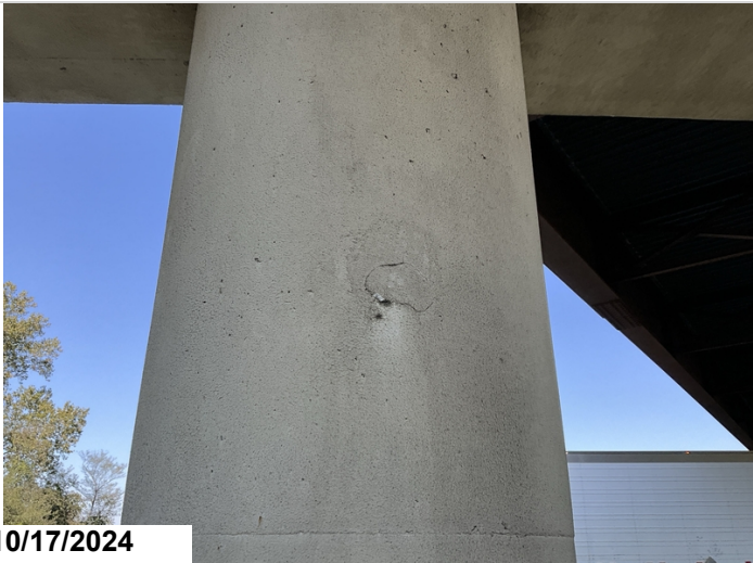
Bent 3, Column 1: Cracking, 1EA CS2.
