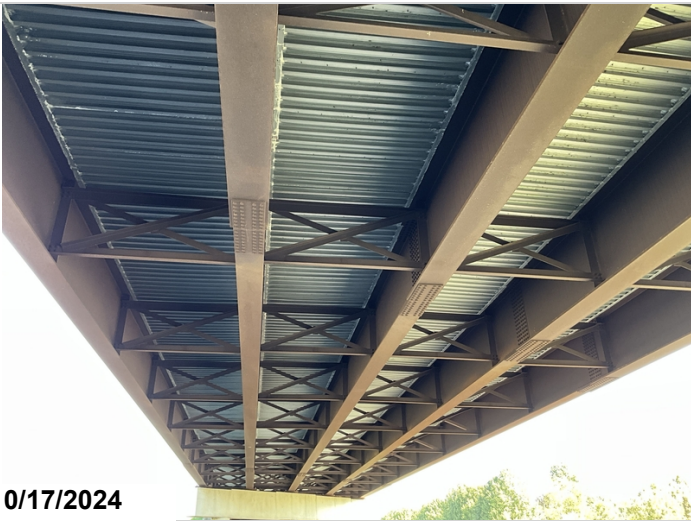
Typical undersurface.
