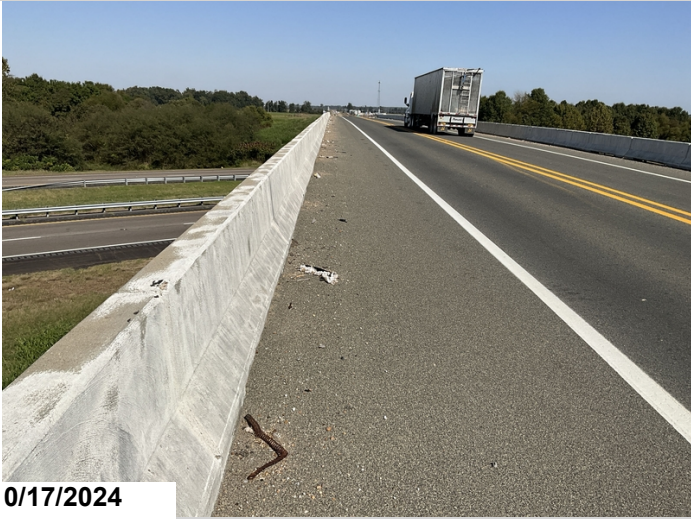
Deck has dirt & debris along gutter lines.
