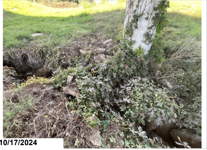
Bent 2, Column 1: Minor erosion around the column, 1EA, CS2.
