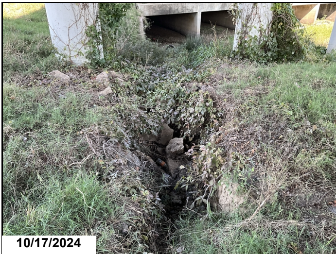
Span 1, Bent 2: Erosion around Column 1.
