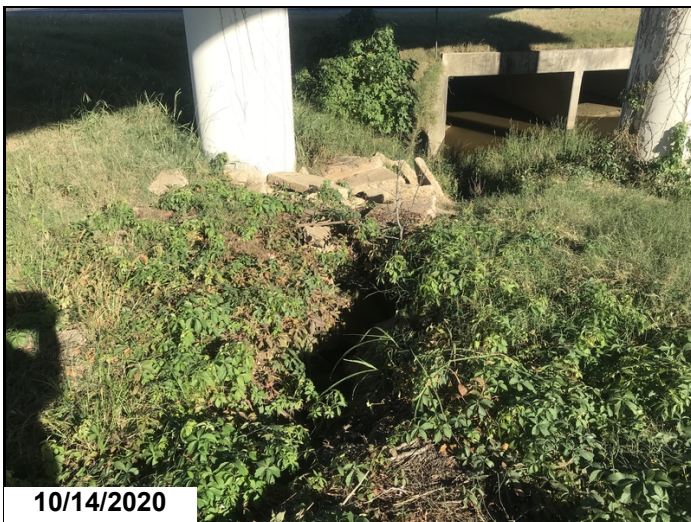
Span #1, near bent #2 column #1 has 3' wide by 3' deep vein of erosion.
