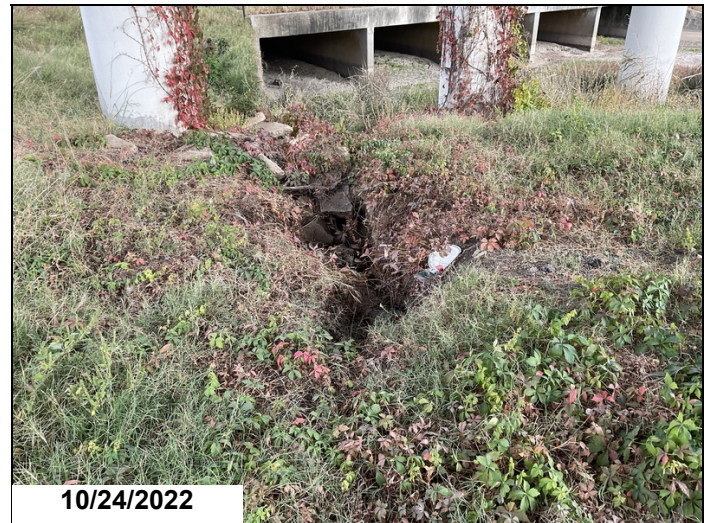
Erosion span #1 near bent #2
