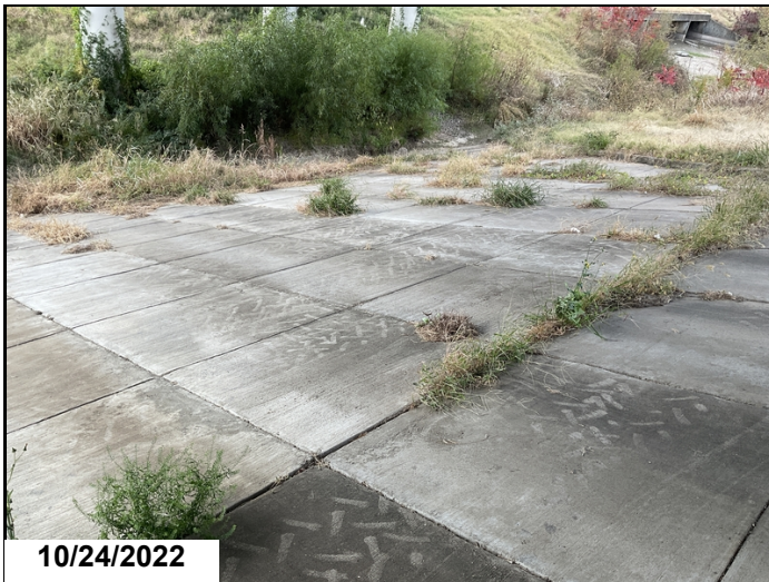
Vegetation growing in slope pavement joints abutment #2
