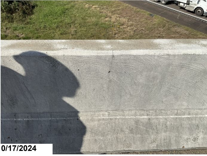
Typical vertical cracking. CS2.
