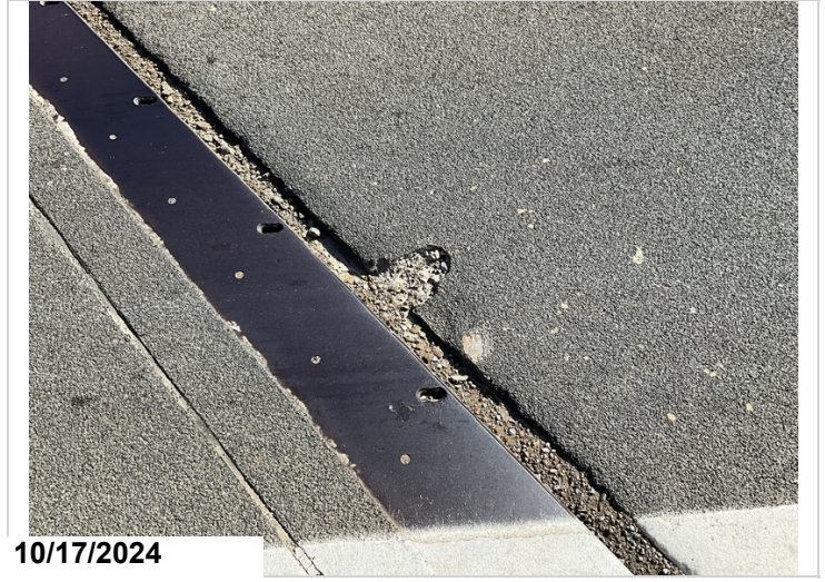
Span 4, Bent 5: Spalling. 1' CS3.
