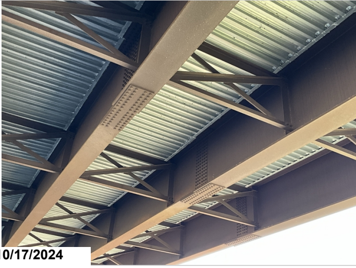
Girders: Typical field splice connections.
