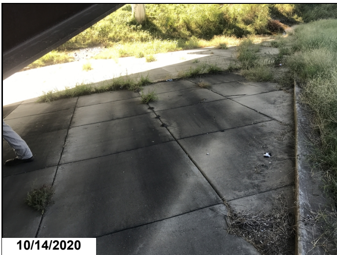
Vegetation growing in slope paving joints.
