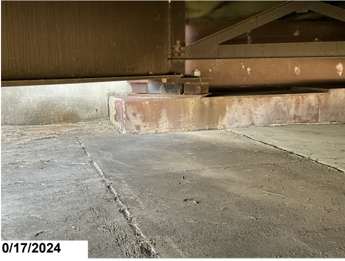
Typical elastomeric bearing.
