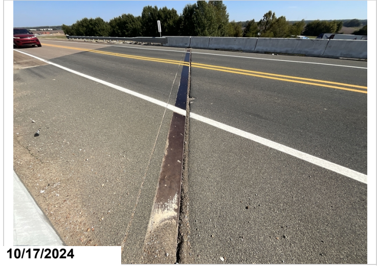
Bent 5, Joint: Debris impaction. 38LF CS2.
