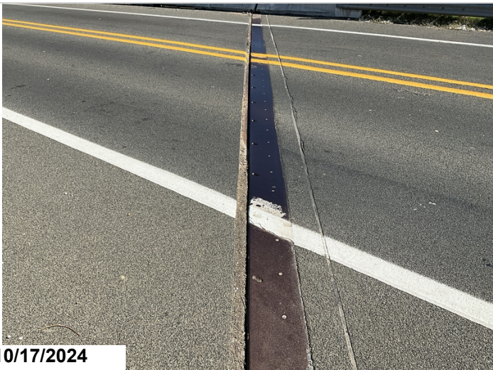
Bent 1, Joint: Debris impaction. 41LF CS2.
