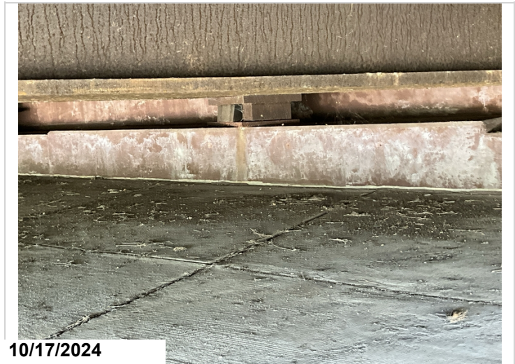
Bent 1, Bearing: Leaning towards Bent 1. 67 degrees on 10/15/2024.
