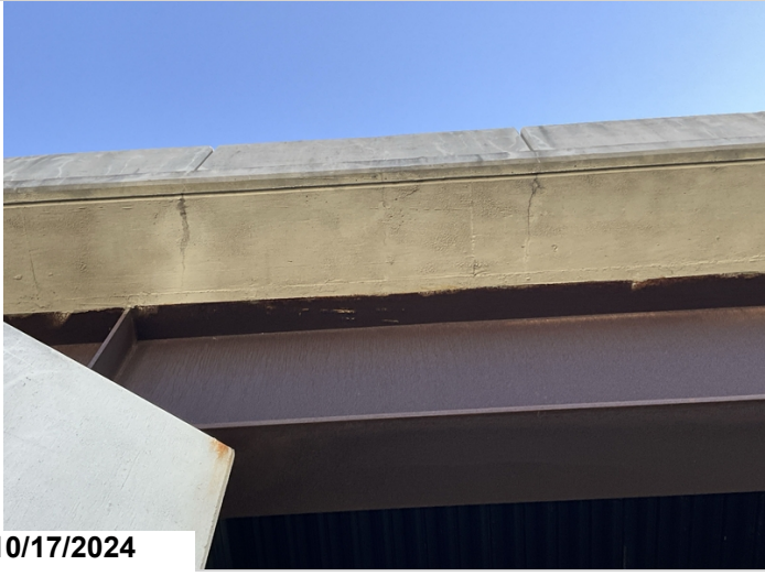
Span 1, Left Overhang: 23 SF CS2 cracking. right 29. Spans 2 & 3, Left Overhang: 47' CS2 Cracking. Right Overhang: 58' CS2 cracking. Span 4, Right: 27'. Left: 32'.
