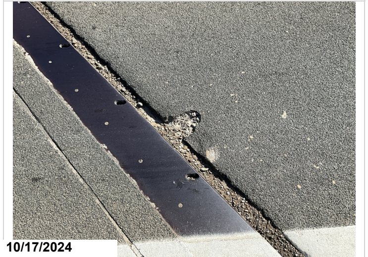
Span 4, Bent 5: Spalling. 1' CS3.
